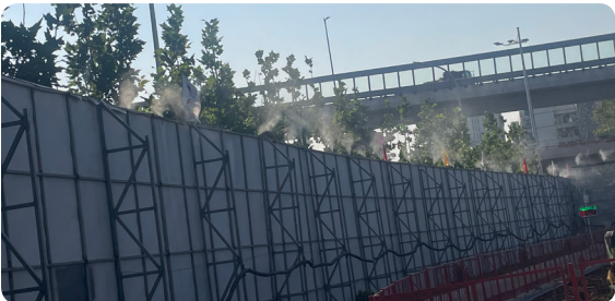
▲ Construction Site Enclosure Sprinkler System
